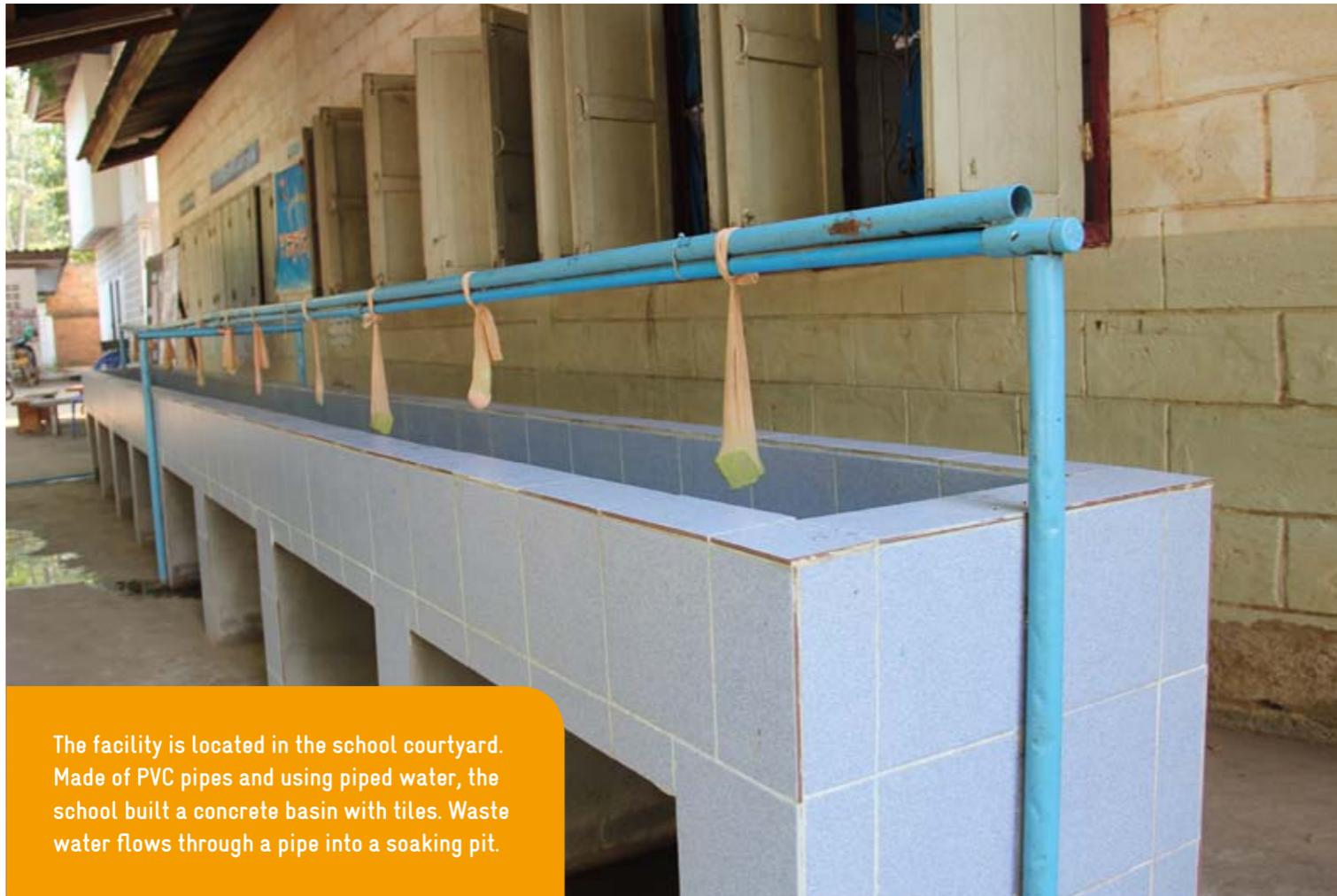
The facility is located in the school courtyard. Made of PVC pipes and using piped water, the school built a concrete basin with tiles. Waste water flows through a pipe into a soaking pit.
