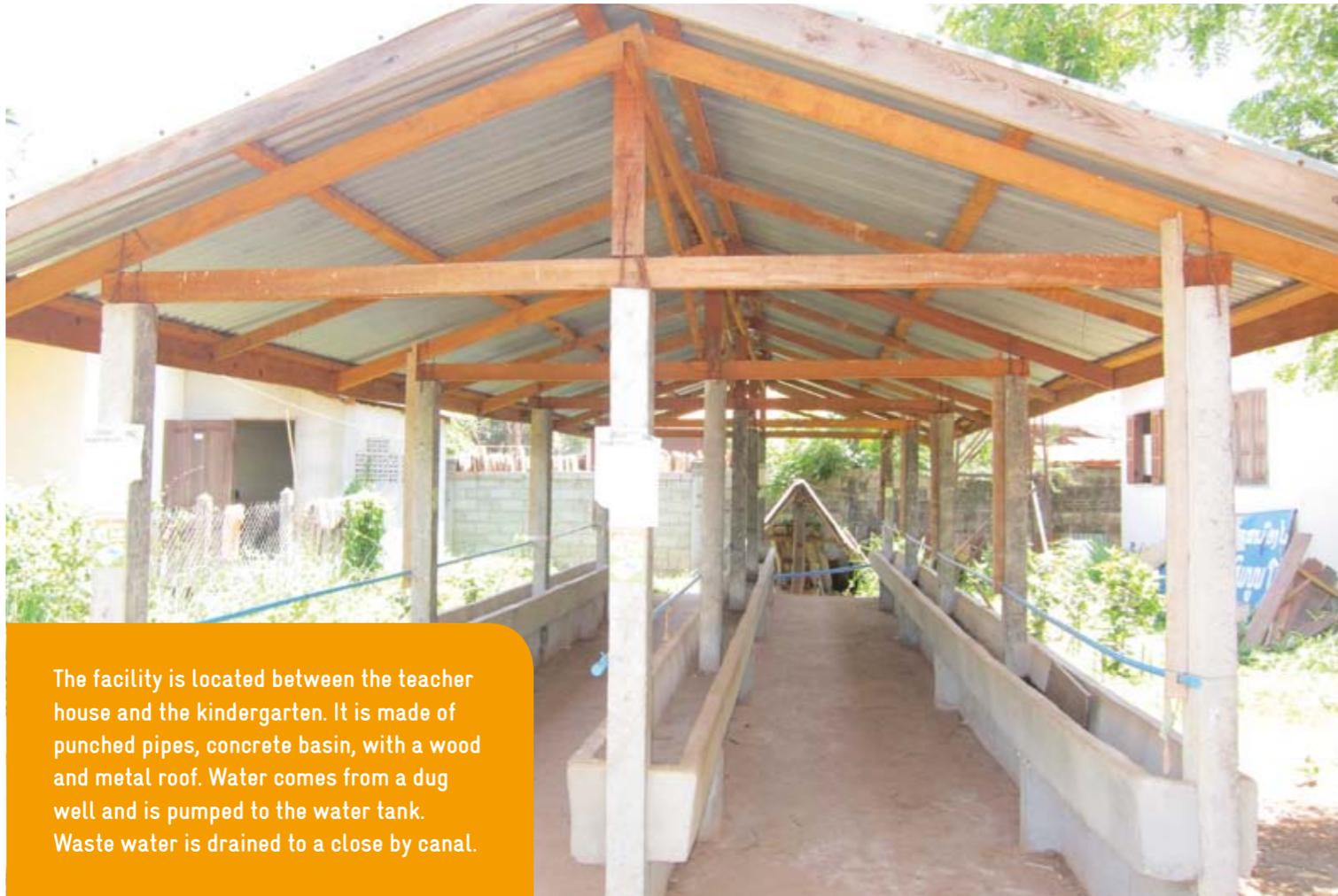
The facility is located between the teacher house and the kindergarten. It is made of punched pipes, concrete basin, with a wood and metal roof. Water comes from a dug well and is pumped to the water tank. Waste water is drained to a close by canal.
