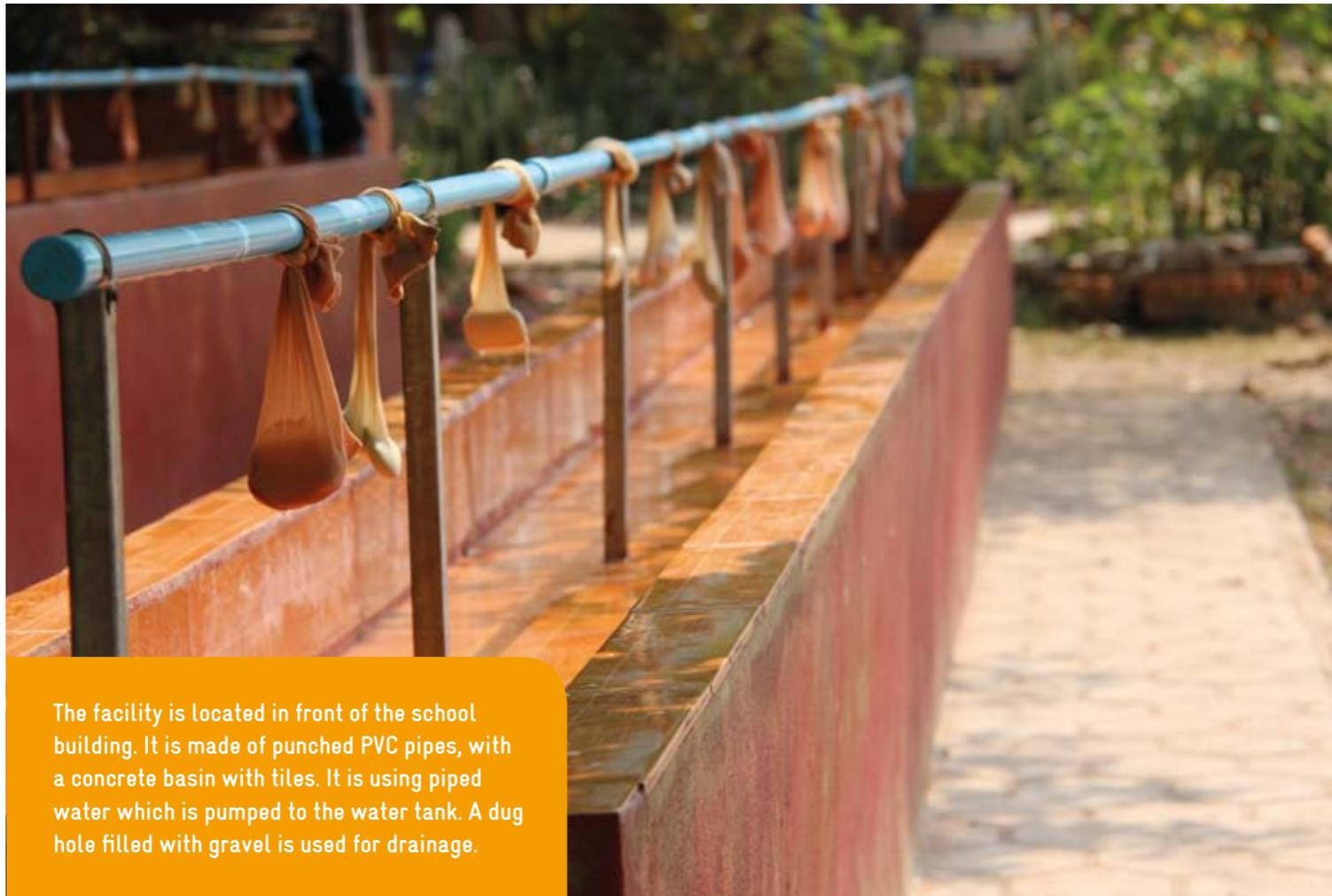
The facility is located in front of the school building. It is made of punched PVC pipes, with a concrete basin with tiles. It is using piped water which is pumped to the water tank. A dug hole filled with gravel is used for drainage.
