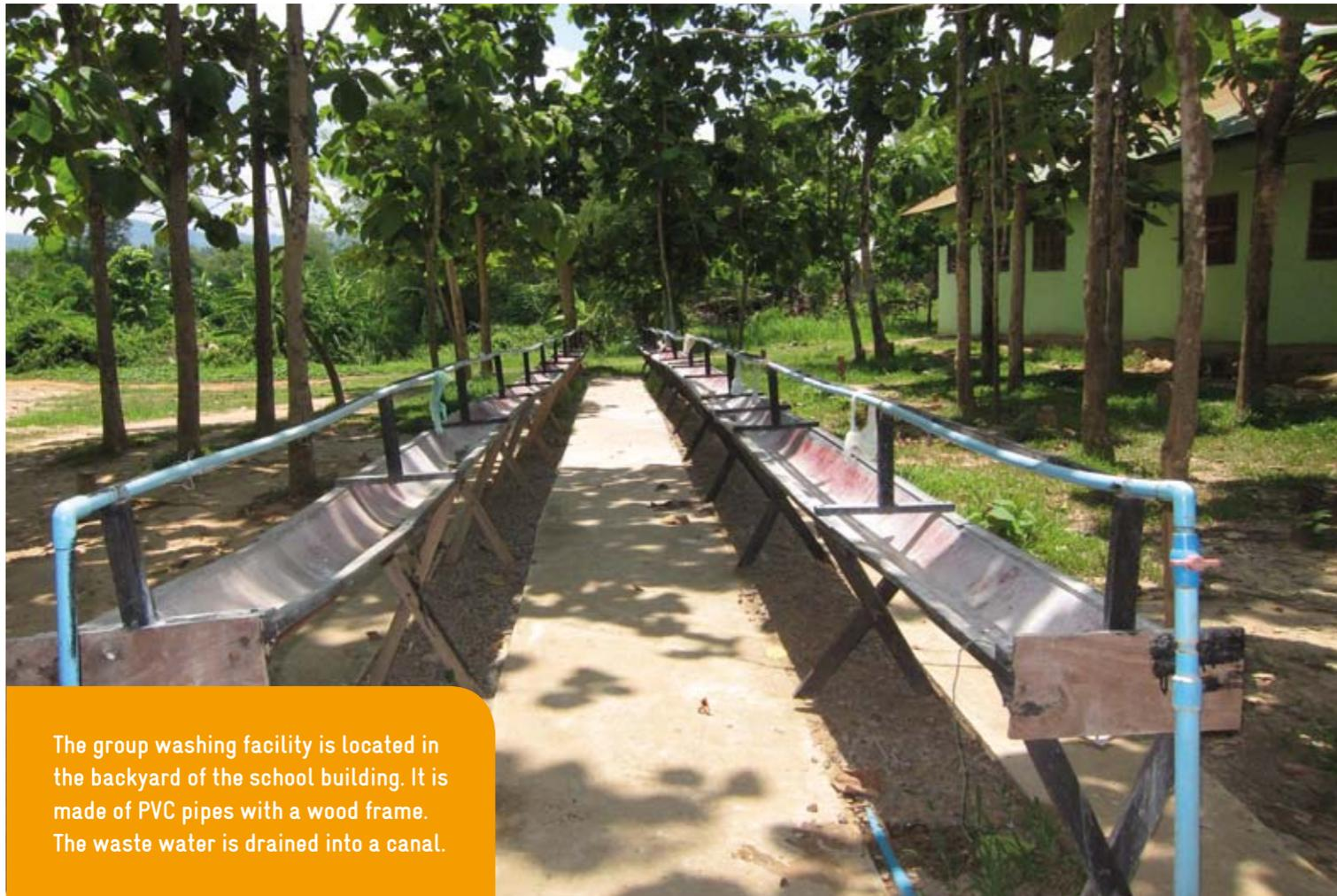
The group washing facility is located in the backyard of the school building. It is made of PVC pipes with a wood frame. The waste water is drained into a canal.
