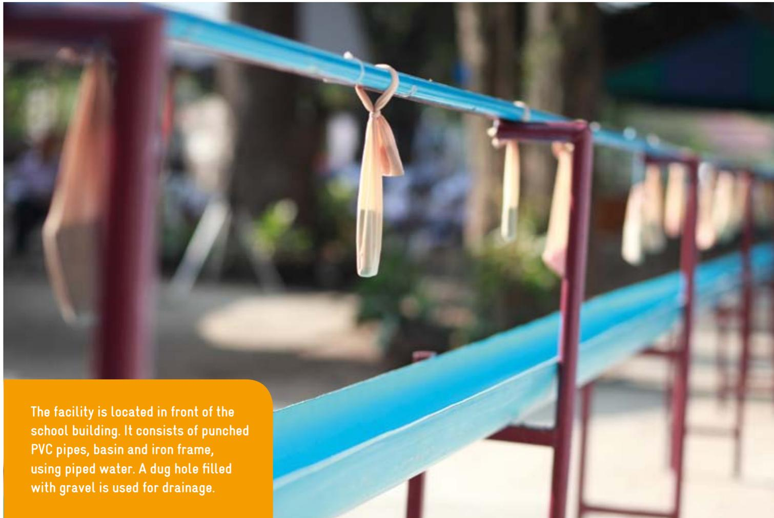
The facility is located in front of the school building. It consists of punched PVC pipes, basin and iron frame, using piped water. A dug hole filled with gravel is used for drainage.
