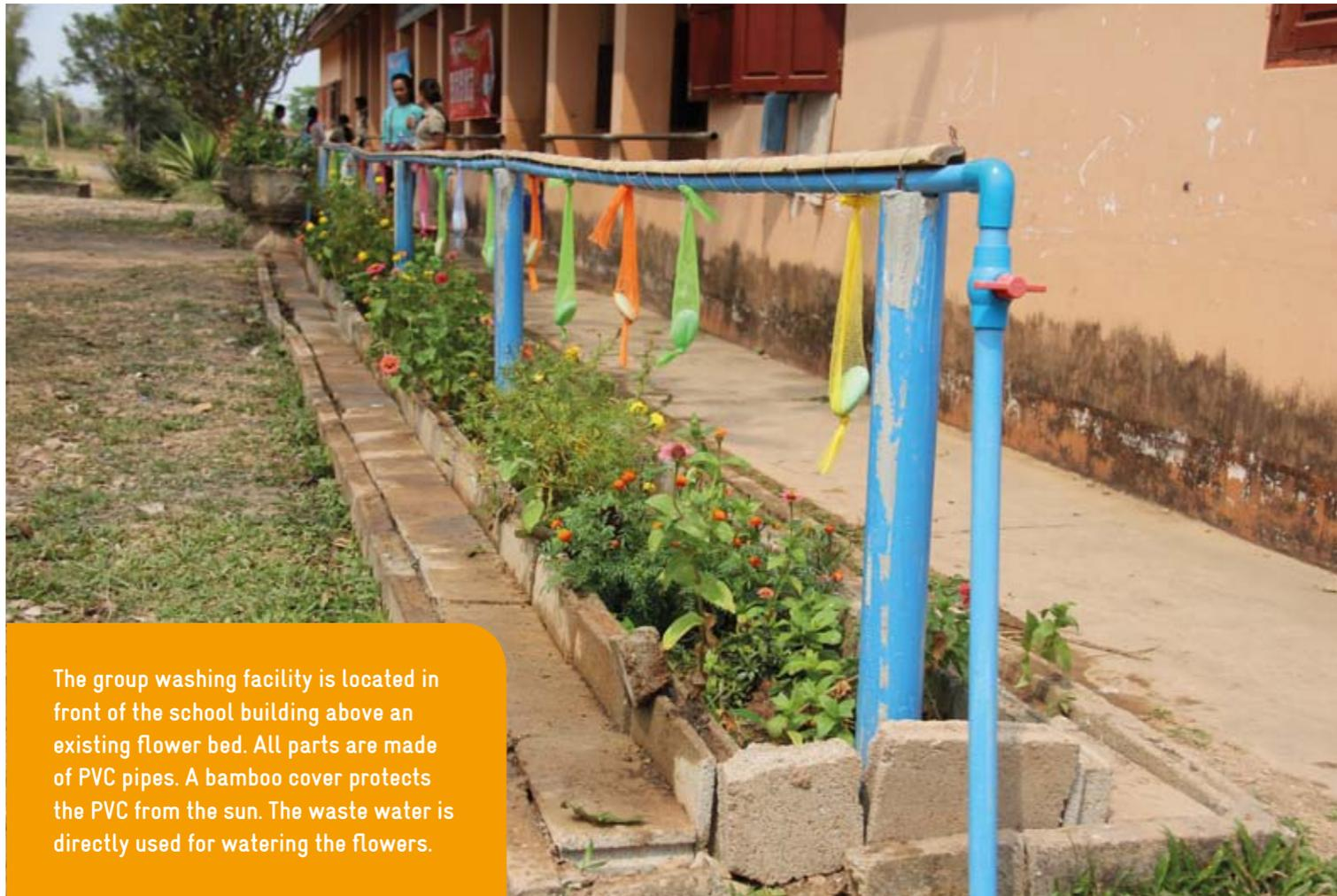
The group washing facility is located in front of the school building above an existing flower bed. All parts are made of PVC pipes. A bamboo cover protects the PVC from the sun. The waste water is directly used for watering the flowers.
