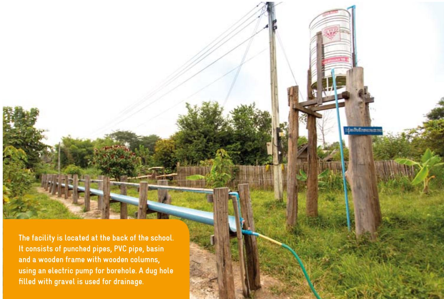
The facility is located at the back of the school. It consists of punched pipes, PVC pipe, basin and a wooden frame with wooden columns, using an electric pump for borehole. A dug hole filled with gravel is used for drainage.
