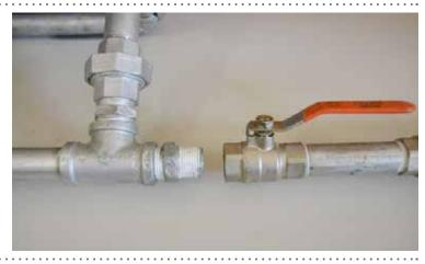
Secure with pipe wrench (Take care that bore holes are pointing straight to the ground).
