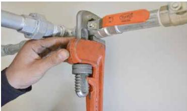
If necessary secure lock nut of valve.
